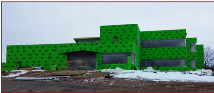
Gateway Ticketing Systems work continues
