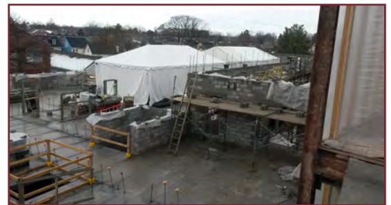
Keystone Villa At Ephrata work continues outside
